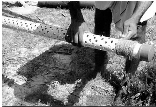
FIGURE- 2 FARMER PREPARING THE PVC PIPE FILTER
